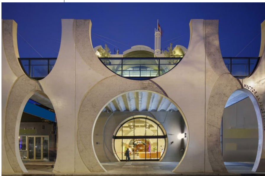
Left: Victorian Pride Centre, 2022. First of its kind in Australia, the Victorian Pride Centre holds, within its 6,200m 2 footprint, symbolic and safe space for members of the LGBTIQ+ communities. High performance glazing and an exposed structure demonstrate sustainability in design, minimising material use and maximising energy efficiency. Photo: John Gollings
